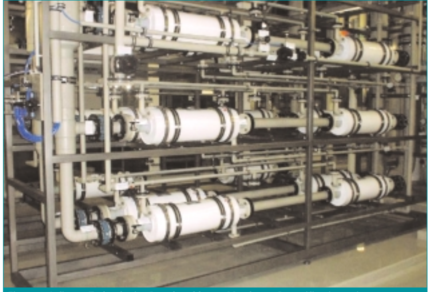
Figure 8. Infineon Technologies Dresden, SC 300: Membrane Degasification units.
